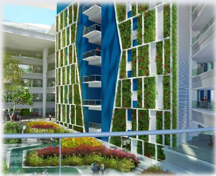
Extensive Green Wall on West Facing Facade
