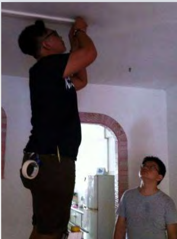
Electrical student s at work installing the light fittings
