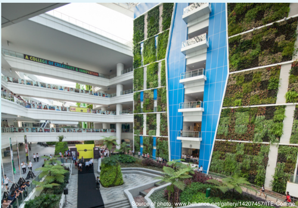
Vertical green walls installed on west-facing facades of building walls at ITE College Central, Ang Mo Kio
