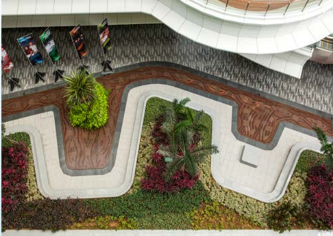
Top view of a section of ITE College Central, Ang Mo Kio
